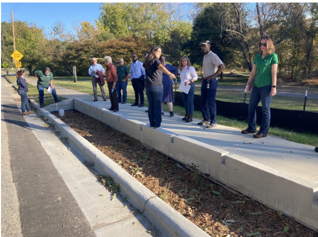
Staff discussing Peterson Street Linear Bioretention Area
