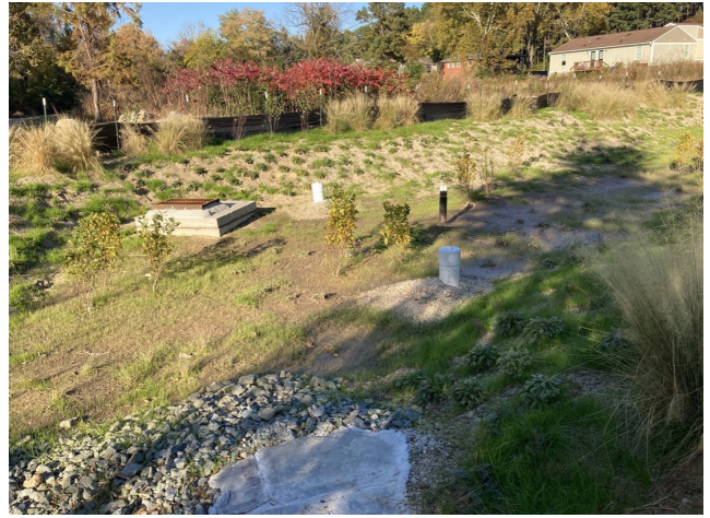
Walnut Creek Gravel Wetland completed in Fall 2021
