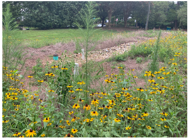
Glen Eden Pilot Park Bioretention Area
