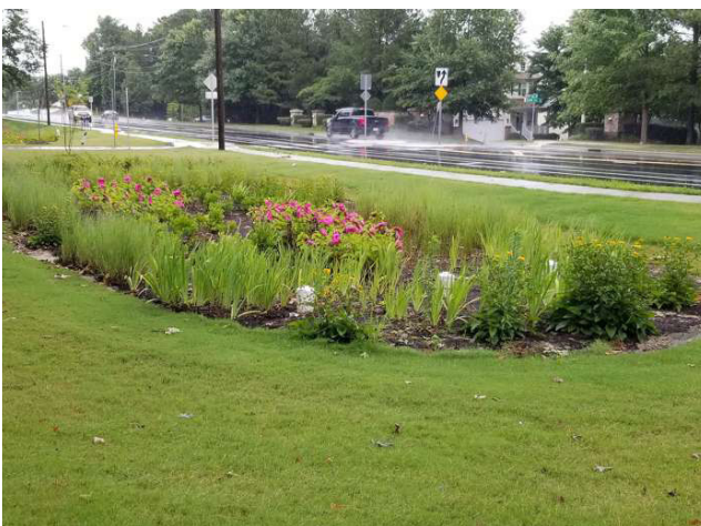
Fox Road Bioretention Area
