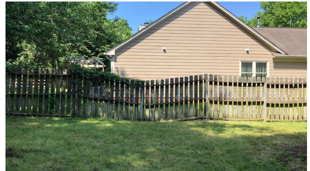
A sinkhole in a yard on Fairlie Place
