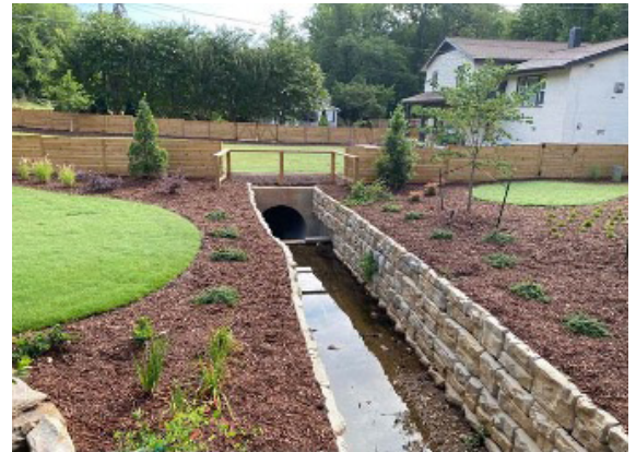
Completed Swann Street Drainage Project
