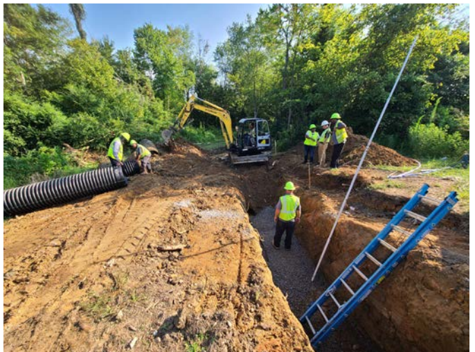
Bailey Drive Construction
