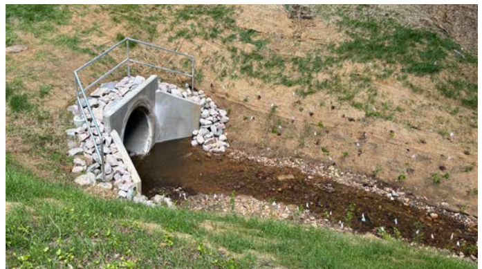
North Hills Drive Headwall Completed
