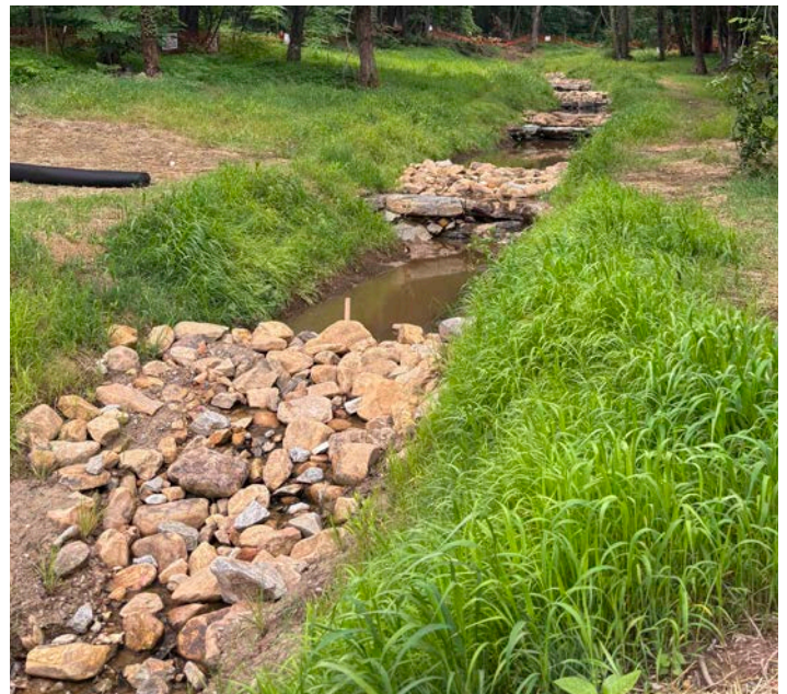
NCMA Stream Restoration
