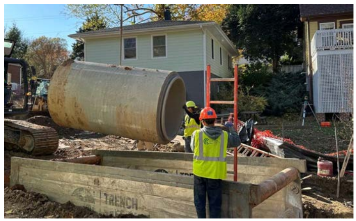
North Boundary Repair
