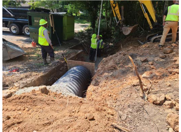
Pullen Park Construction
