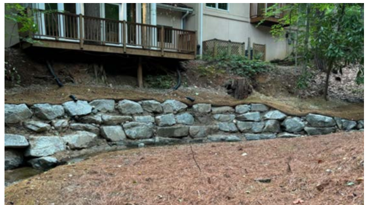
Northbrook Drive Stream Repair
