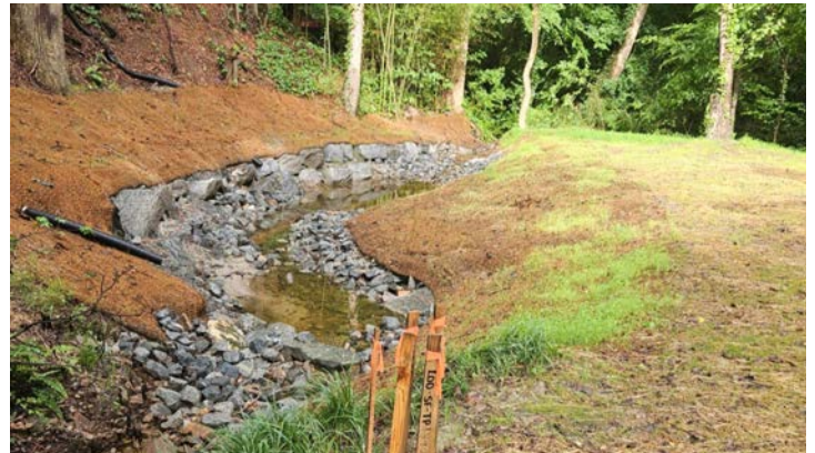
Hunting Ridge Stream Repair
