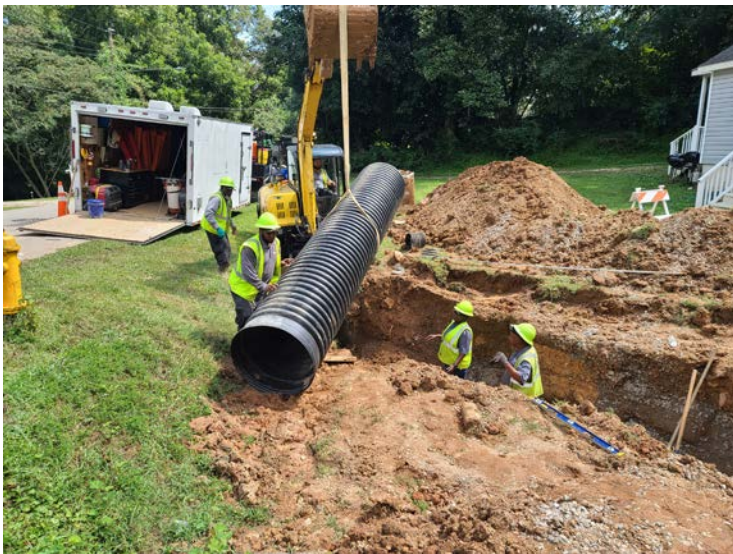
Steel Street Construction
