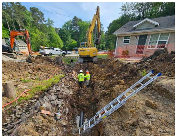
Construction at Glenbrook Dr and Dacian Rd
