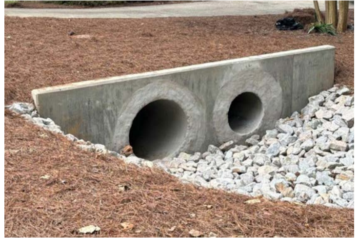
Dresden Lane Replaced Pipe
