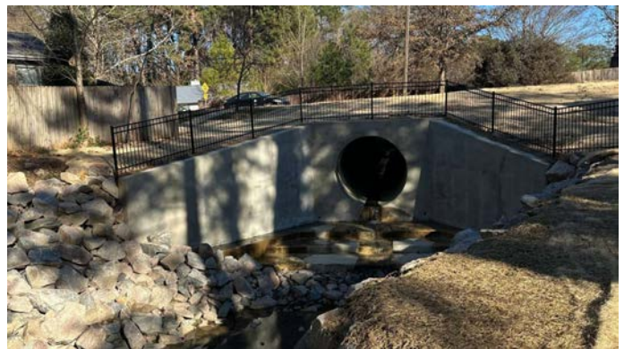
Saratoga Drive Endwall Completed
