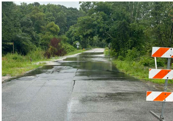
Rose Lane Street Flooding
