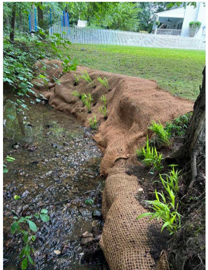
Small-Scale Stream Repair
