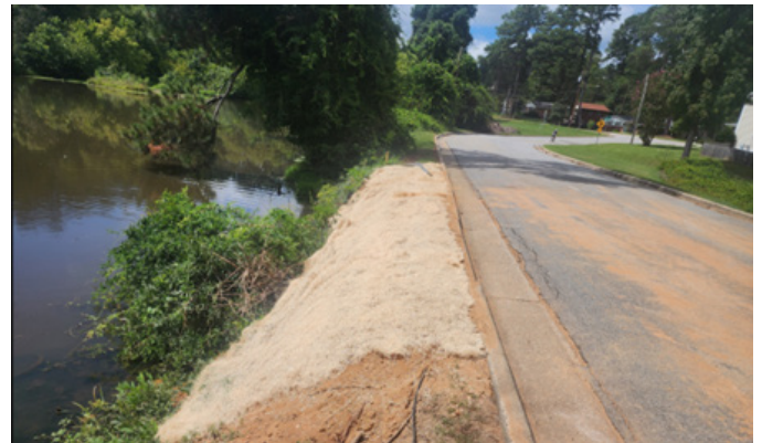
Upper Longview Construction and Completion
