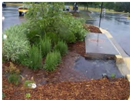
**Figure 3** Example barrier: curb cuts, needed to drain water to GI/LID, are not allowed
