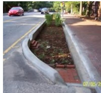
**Figure 2** Pullen Road Curbside Planter Box/Bioretention
