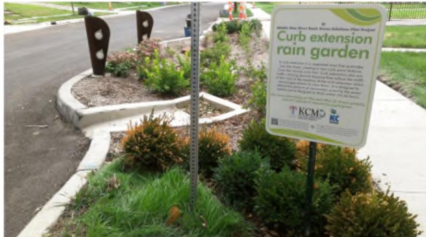
Figure 7 roadside Bioretention
