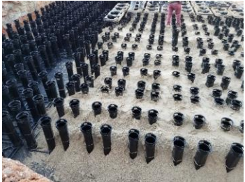
Underground View of Suspended Pavement
