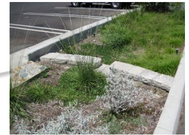
Check Dam Example
