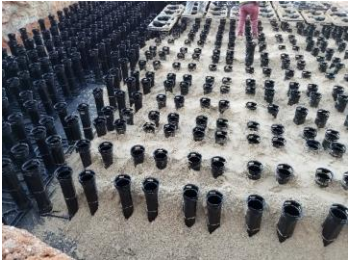
Underground View of Suspended Pavement
