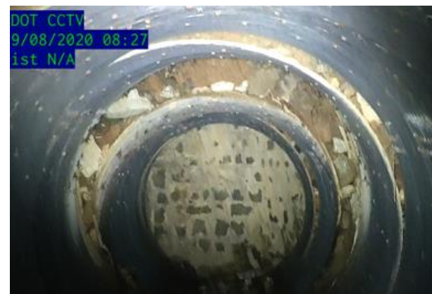
Offset pipe joints
