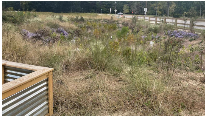
Example of a completed subsurface gravel wetland on Peterson Street across from the Walnut Creek Wetland Center and the Little Rock Greenway Trail.
