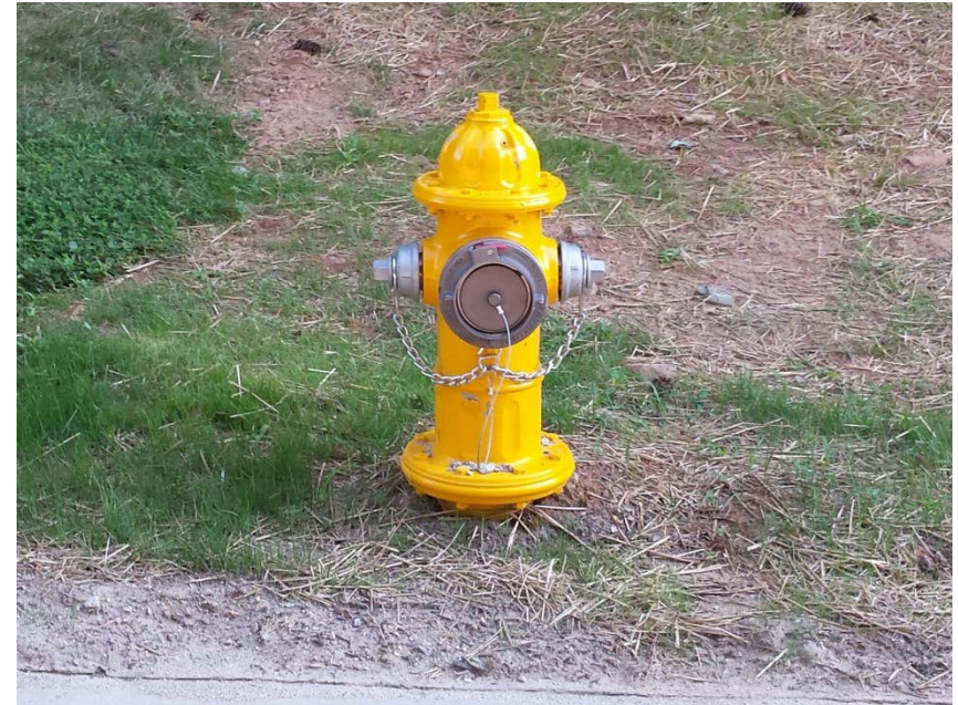
New Fire Hydrants
