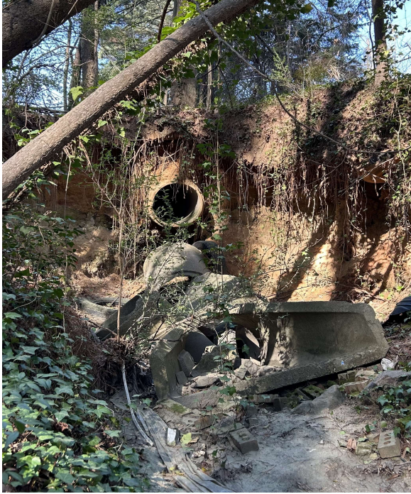
Photo 1-5 Example of Stormwater Infrastructure with a High Condition Assessment Score
