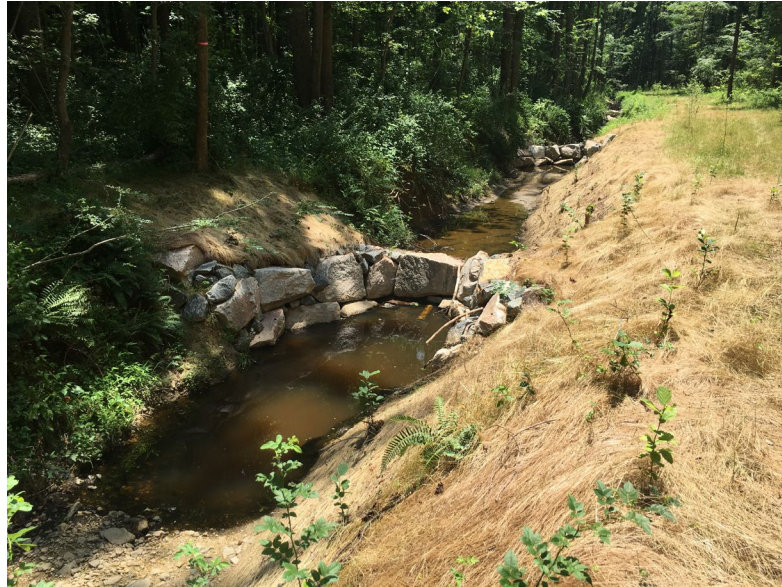
Post-construction in-stream structure 2019
