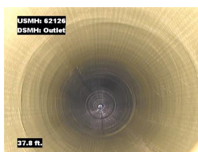
Projects to renew poor condition pipes (left) using trenchless lining techniques (right) are underway
