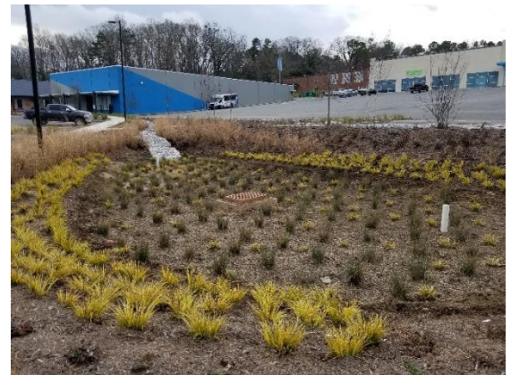
Bioretention Area to Treat Runoff at Gateway Plaza
