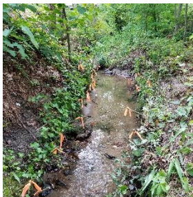
Live Plant Stakes Installed near Marshall Street for Stream Bank Stabilization
