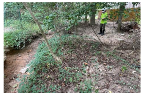
Farther upstream on same ditch, near fence line at 9420 Waterwood Ct. (facing SE)
