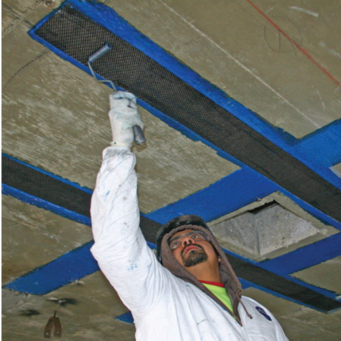
Carbon Fiber Wrap Installation
