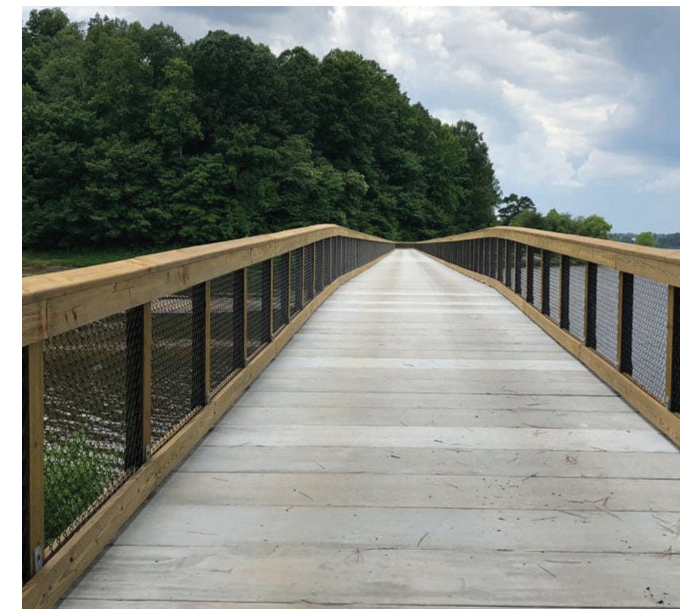
Boardwalk with wood and metal railing
