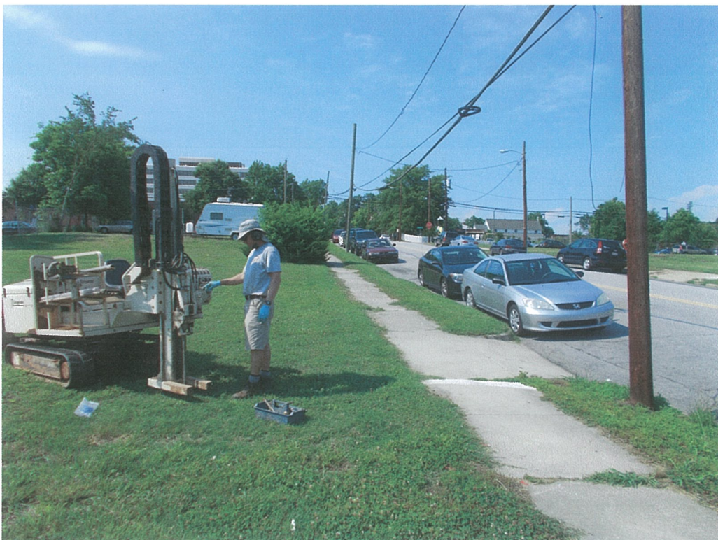
Geoprobe at Location of Sample No. GW-6 Eastern Property Boundary Near S. Bloodworth Street
