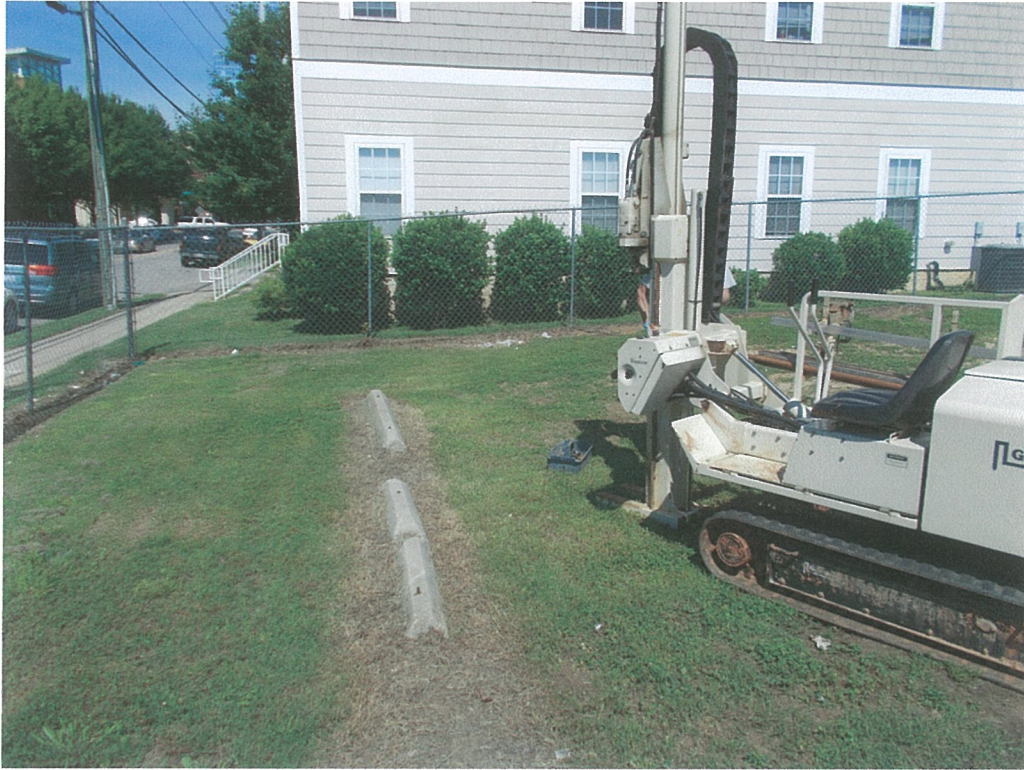
Geoprobe at Location of Sample Nos. GW-1 and S-1 Southwest Corner of Subject Property
