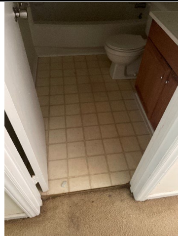
Off-White Vinyl Flooring- Unit C Bathroom
