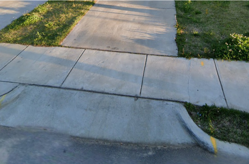
TOP Sidewalk detail over residential driveways
