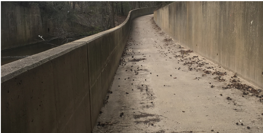
Shown is the channelized portion of Walnut Creek with concrete trail and retaining wall. This portion of the trail occurs by South Saunders Street.
