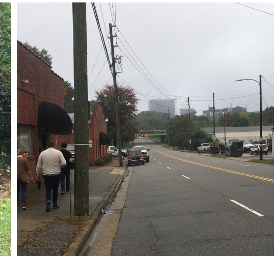
Commercial areas have poor sidewalk conditions.
