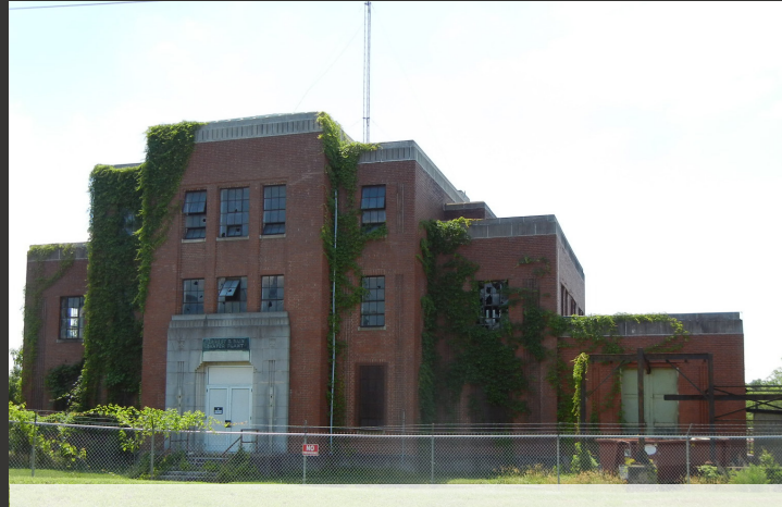
The E.B. Bain Water Treatment Plant is a designated Raleigh Historic Landmark. In operation from 1940-1987, it was used as storage until 2006 when purchased by Empire Properties.
