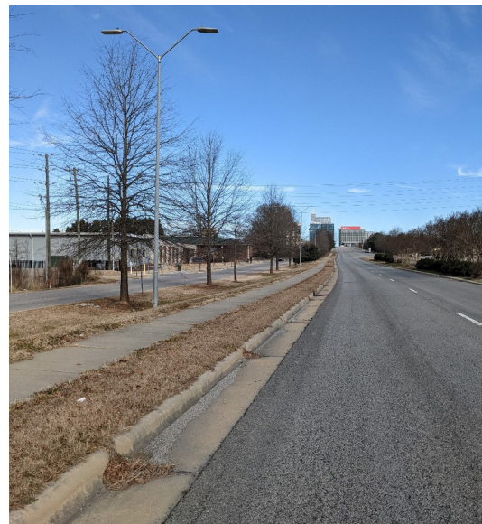
LEFT Sidewalk facing northbound on S. Wilmington Street at City Farm Road
