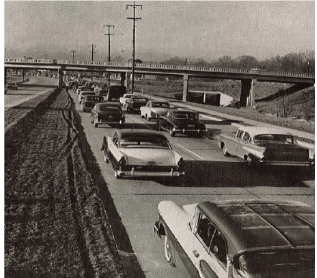
Capital Boulevard (shown) and the Beltline facilitated auto-oriented development on the city's edges
