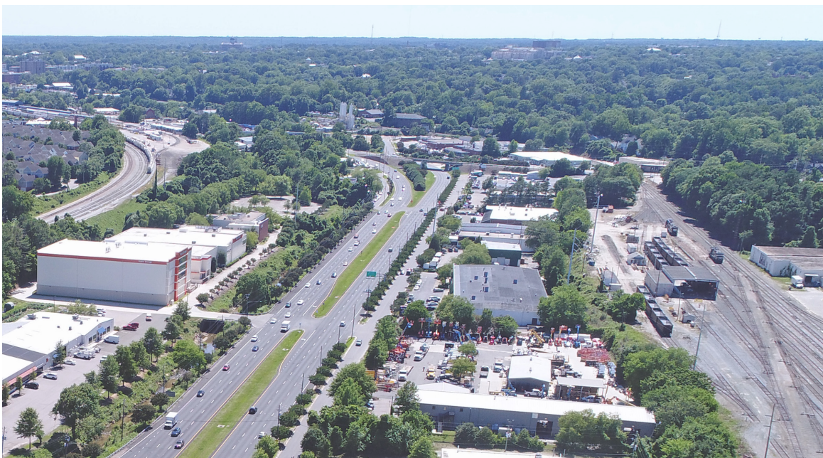
Industrial uses line the northern corridor along Capital Boulevard.
