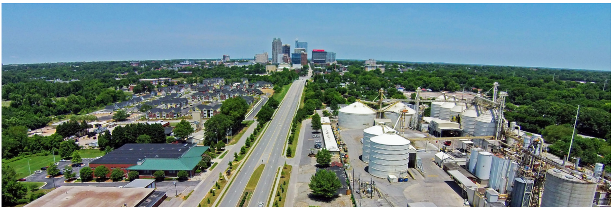
Land acquisition along the corridors, such as along S. Wilmington Street (shown above) can facilitate the creation of long-term affordable units
