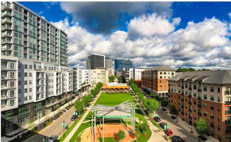
Higher density development transitions to lower buildings to connect to lower density districts
