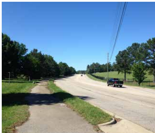
The section of Falls of Neuse Road between Durant Road and Raven Ridge Road currently has a multi-use path on the east side. A sidewalk should be added to the west side of the road, and streetlights added where currently not present.
