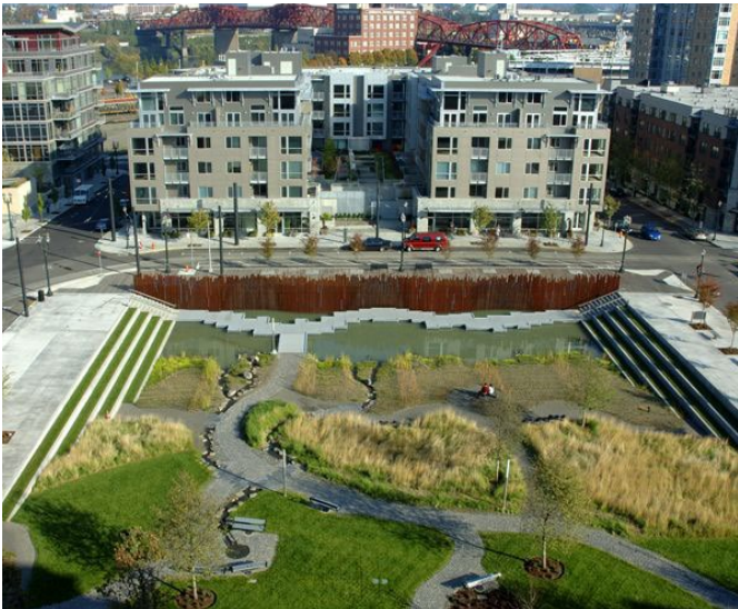
▲ Tanner Springs Park in Portland, OR. Active/passive spaces are layered on top of rainwater infiltration and detention wetlands.
