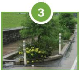
Stormwater Bump-outs
