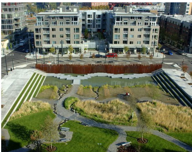
Tanner Springs Park in Portland. Active/passive spaces layered on top of rainwater infiltration and detention wetlands.
