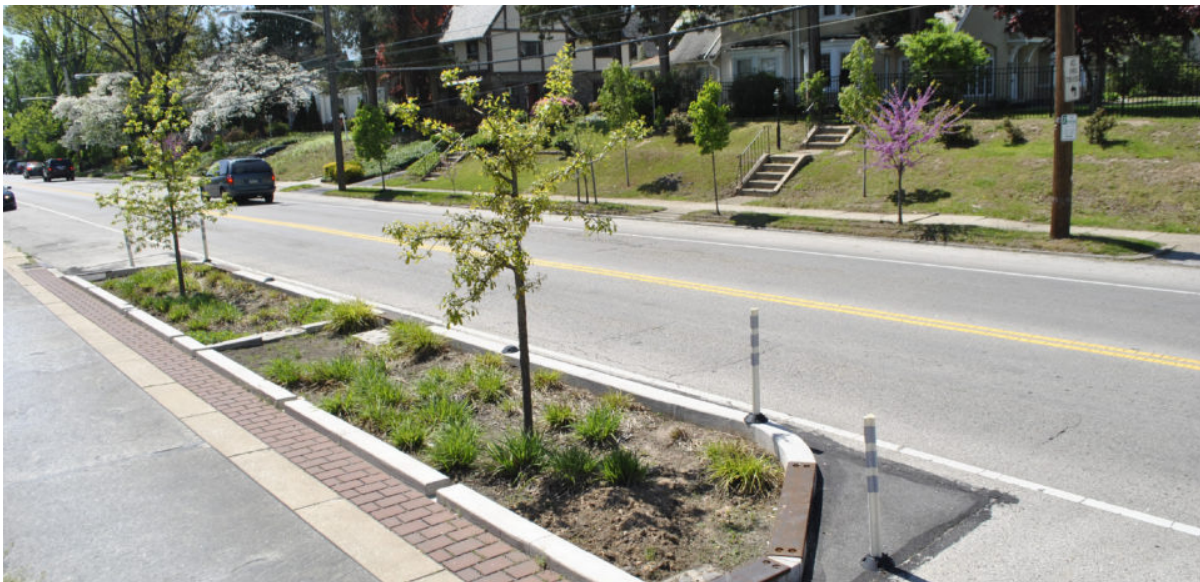
Example of a stormwater bump-out that could be included in a Green Street.
