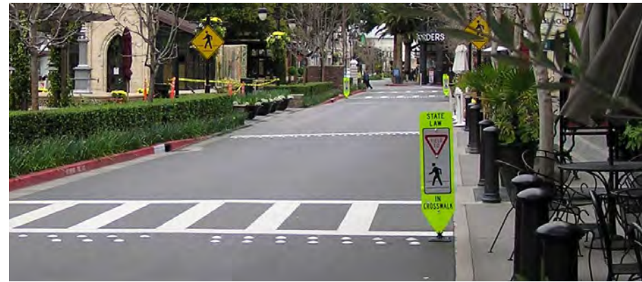
Typical High Visibility Crosswalk with Reflectors and Signs
