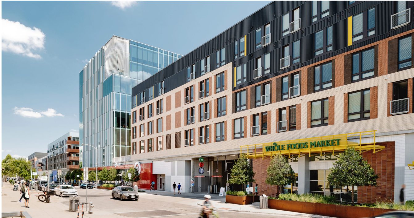
Block A of Plaza Saltillo includes a concrete podium that integrates a grocery store and parking under the residential portion of the building.
