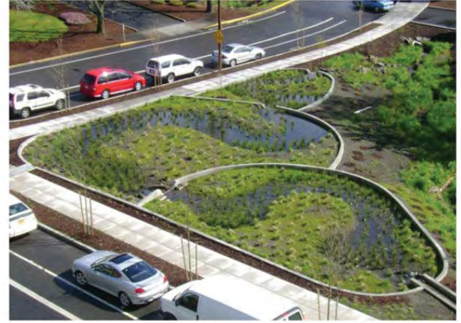
This bioretention facility took the place of an asphalt parking lot that routinely flooded. The install was part of Portland's Green Street Program. Source: Streetsblog San Francisco
