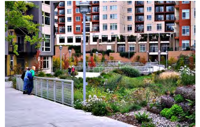
This bioretention facility took the place of an asphalt parking lot that routinely flooded. The install was part of Portland's Green Street Program. Source: Streetsblog San Francisco
