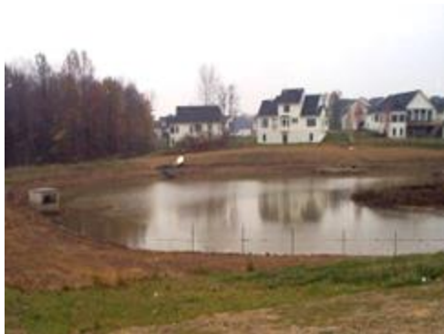
Typical Centralized Detention Pond
