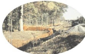
5. Erosion & Sediment Control
