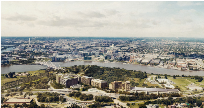
COLUMBIAN QUARTER WASHINGTON, DC REVITALIZED COMMUNITY IN A TRANSIT-ORIENTED DISTRICT | 15-MINUTE NEIGHBORHOOD
