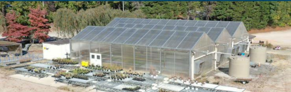
Raleigh Rainwater Rewards (R3) Cisterns at Marsh Creek Park Greenhouse
