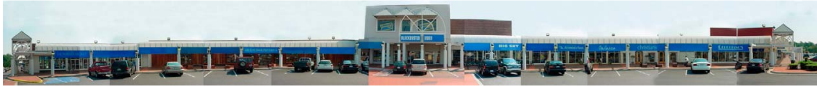
North Elevation - Cameron Street
