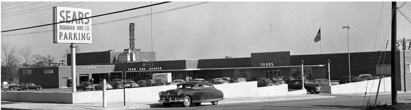
This image demonstrates a historic precedent for High Profile Ground Signs at "Cameron Village". The Village District will NOT allow the use of ground signs of medium and high-profile classification.
