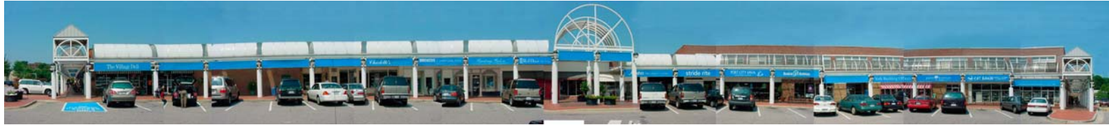
Block 5 South Elevation - Cameron Street
