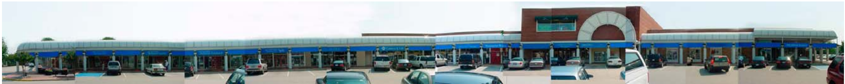
Block 3 West Elevation - Woodburn Road
