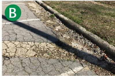
*Buckled and cracked asphalt in parking lot*
