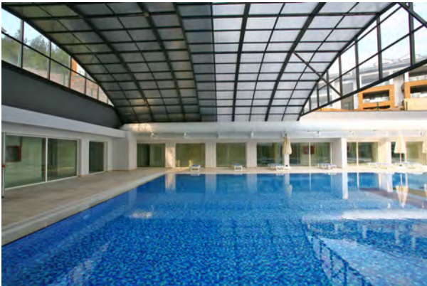
Antorman Complex, Istanbul, Turkey, view of operable roof in open position
