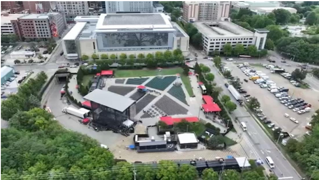
Current location of RHA. Site to the right shows new location and adjacency to the parking deck. Image courtesy WTVD.
