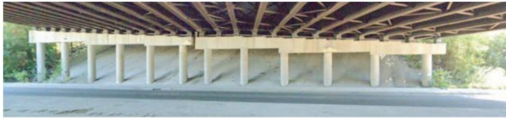
I-40 Underpass Along 401 (Top to Bottom)
