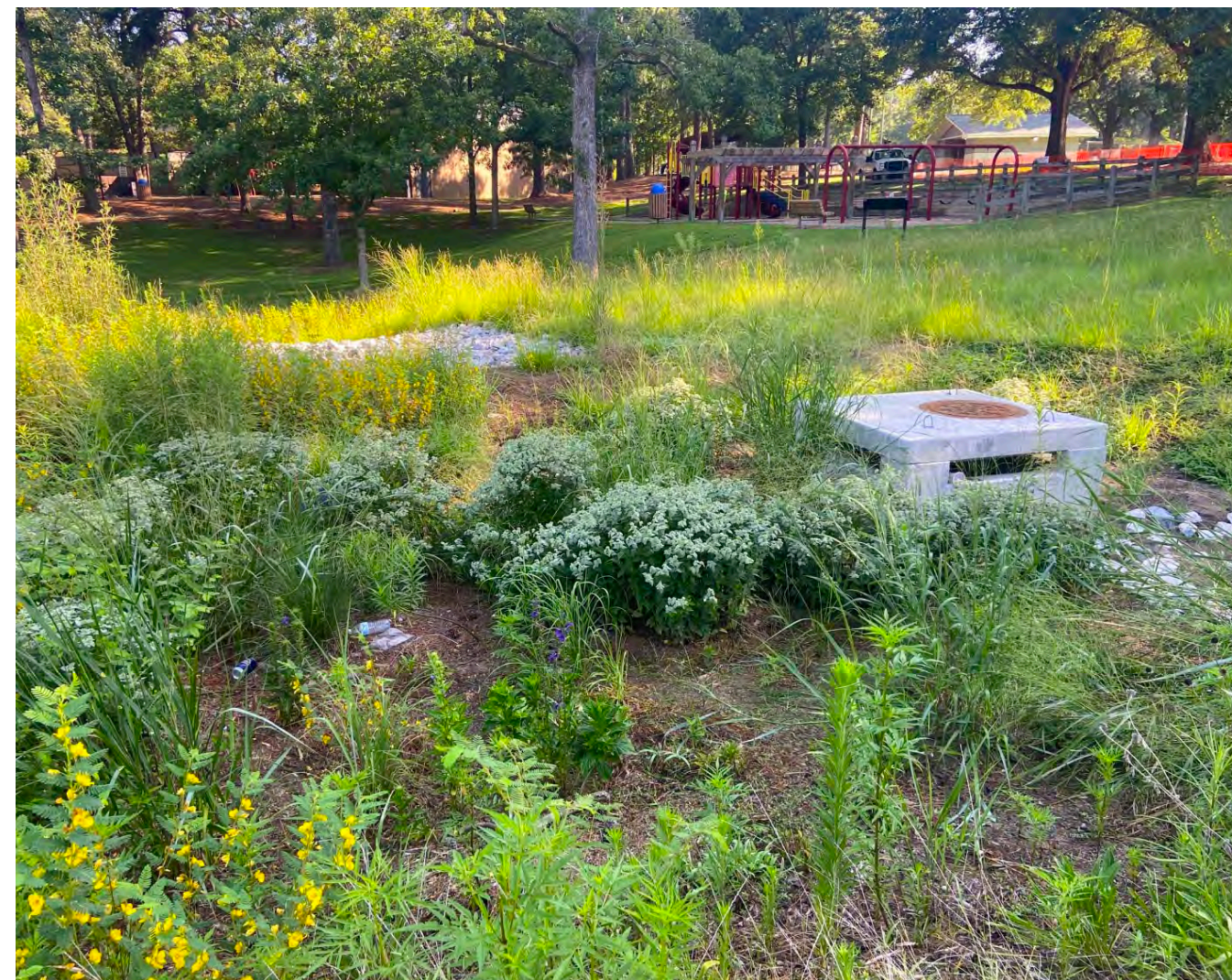
Existing GSI Constructed at Biltmore Hills Park adjacent to Existing Playground and Pool
