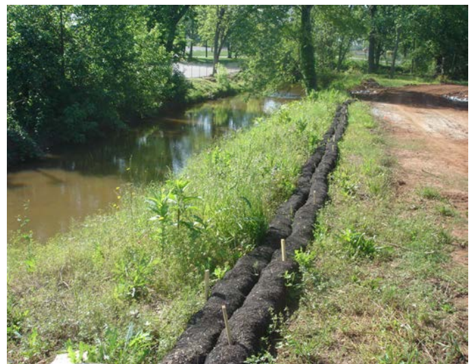
Example of a silt sock controlling drainage along a riparian greenway trail corridor
