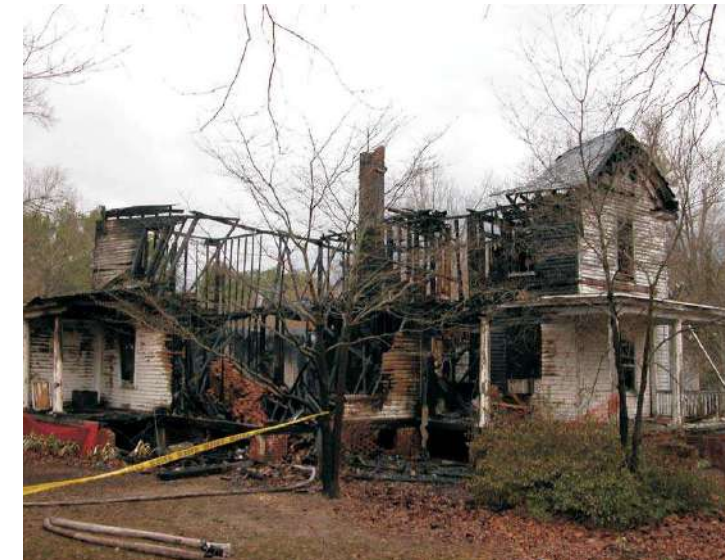
Latta House destroyed by fire Photo Credit: Lloyd Jacobs, Raleigh Historic Landmark Designation Application
