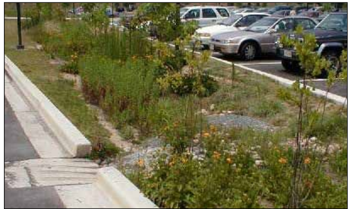
An example of LID / bio-retention stormwater treatment in a parking lot.
