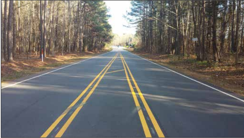
Looking east along Leesville Road. The park property is on the left.
