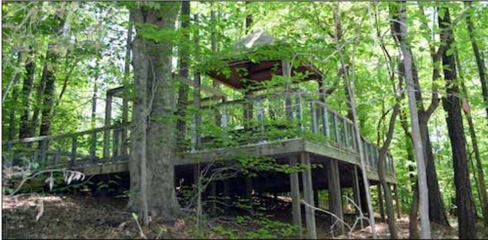
Platform decks at Brookhaven Park in Raleigh.
