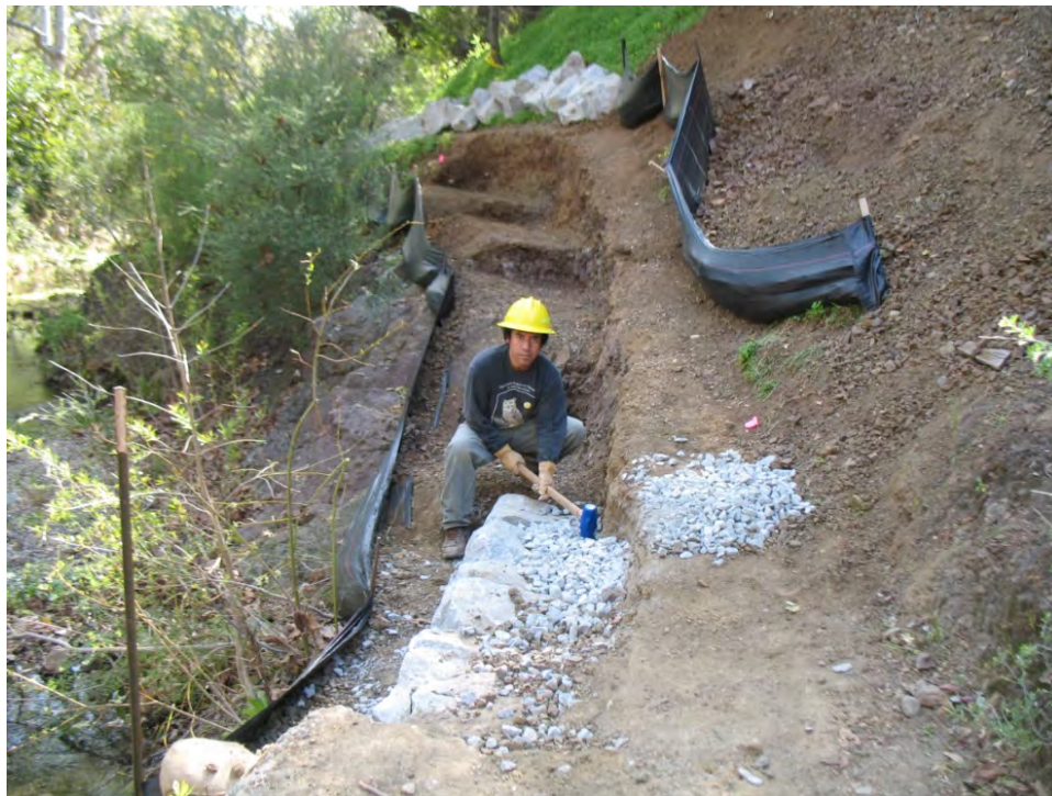
Photo 27.5 - Silt Fence Retaining Soil Above and Below Work Area
