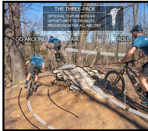
Constructed Rock Kicker with Ride Around
