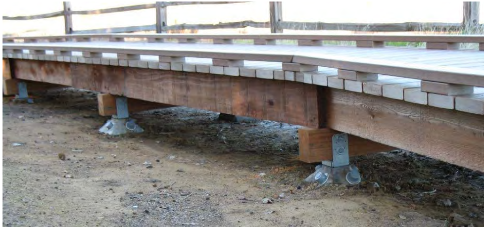
Photo 15.4 - Diamond Pier Boardwalk
