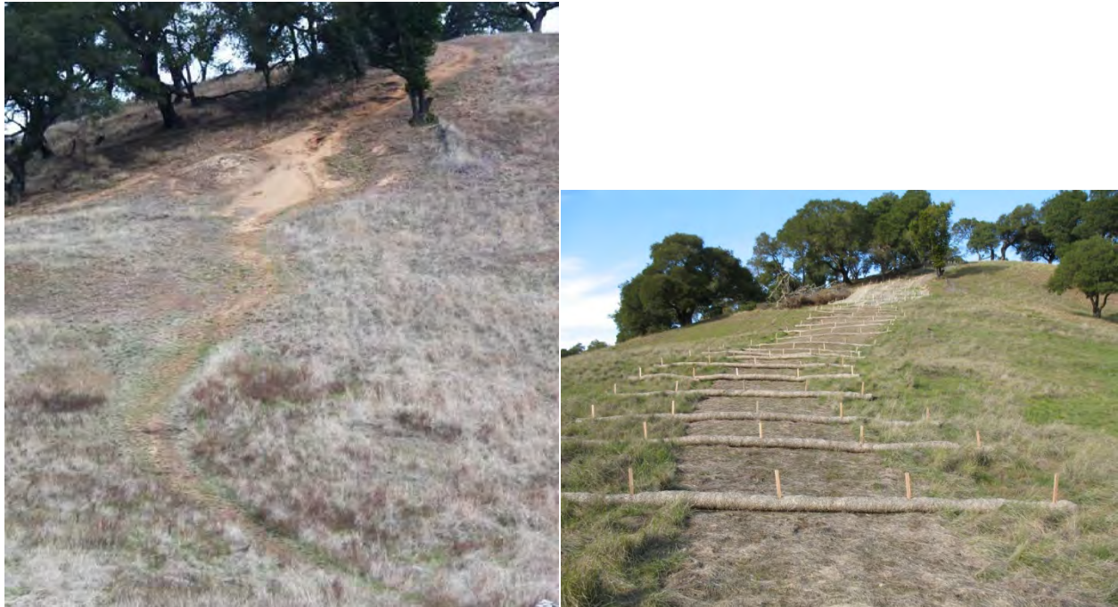
Photo 27.15 - Fall Line Volunteer Trail Restoration Before (left) and After (right)
