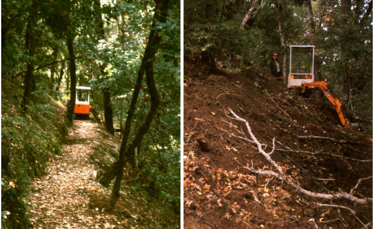
Photo 27.7 - Mini Excavator Recontouring a Trail Prism
