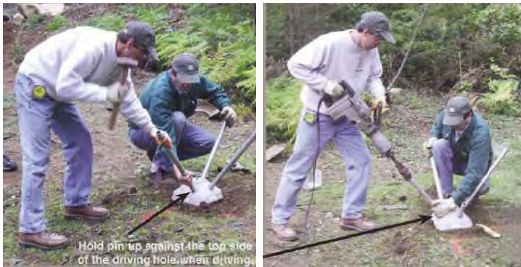
Photo 15.5 - Driving in a Diamond Pier Pin
