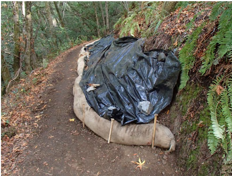
Photo 27.3 - Excavated Soil Retained by Straw Wattles and Covered to Protected from Erosion
