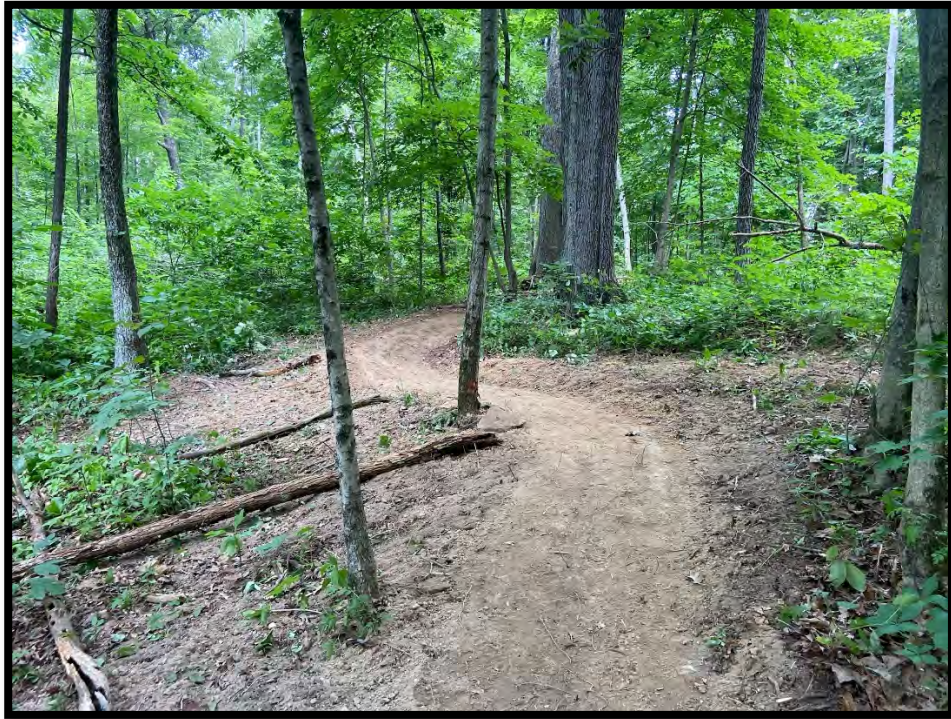
Figure 5: Conceptual experience representing Benchcut Tread construction.
