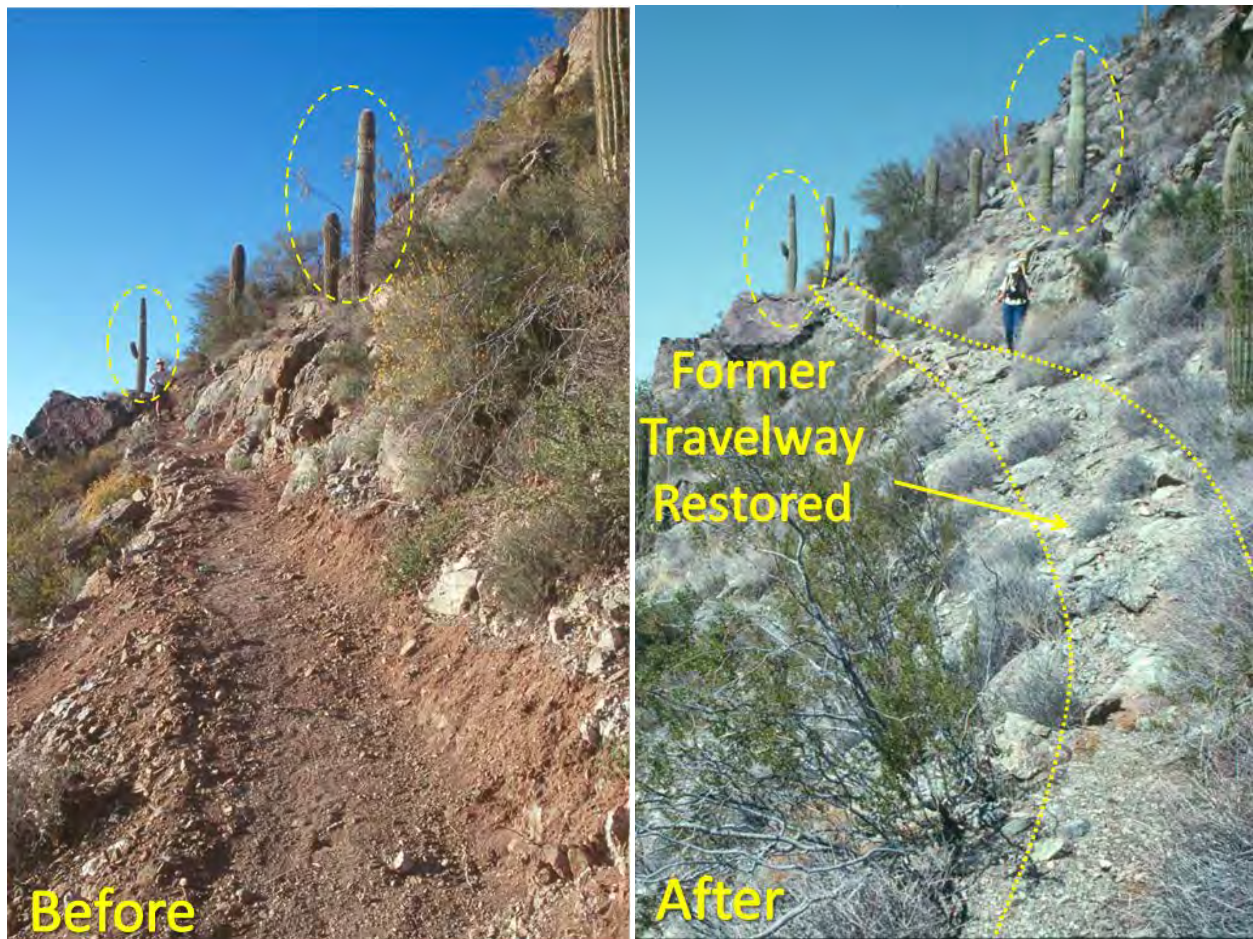
Photo 27.12 - Trail Removal and Recontour Project in the Desert
