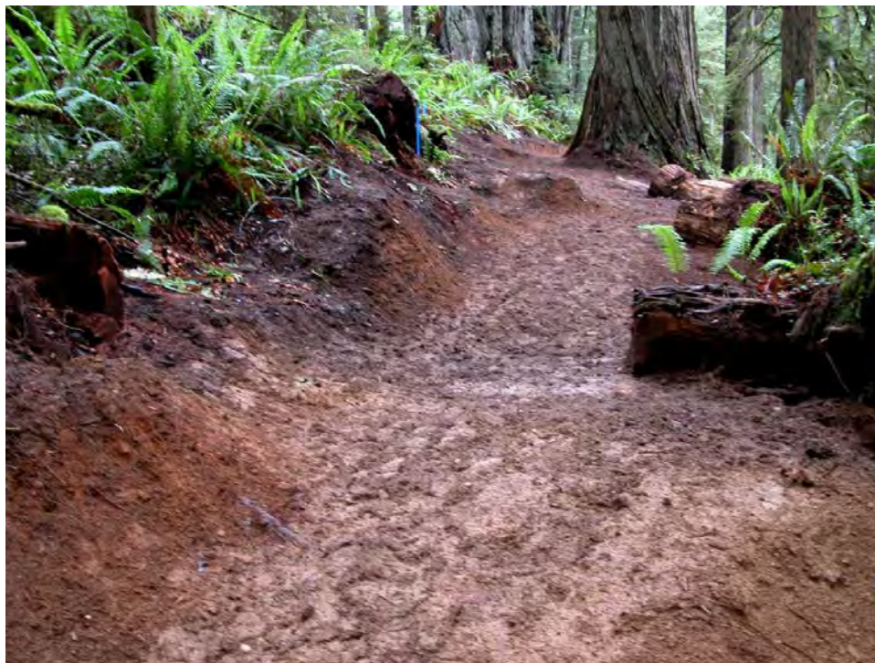
Photo 27.1 - Tread Excavation When Soil is Very Wet
