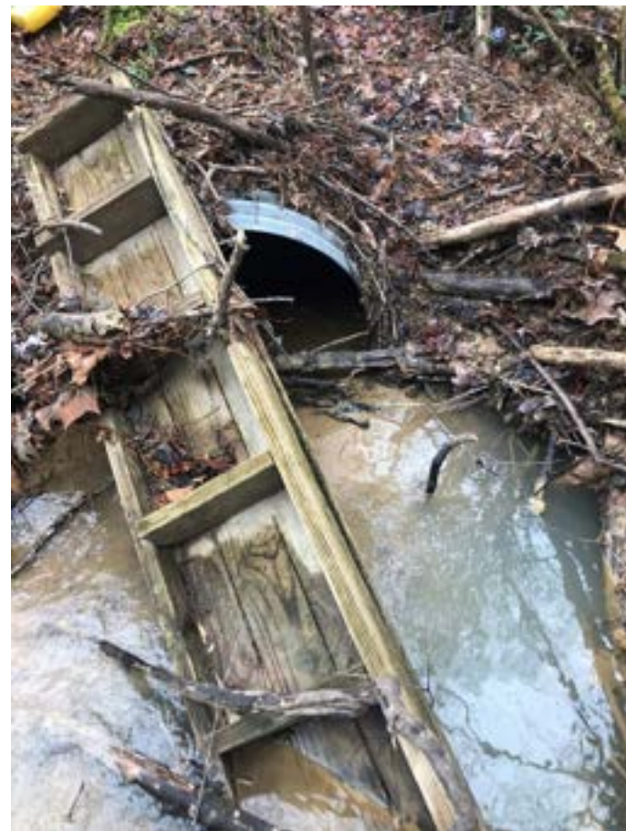
Culvert under Oak Hill Drive roadbed
