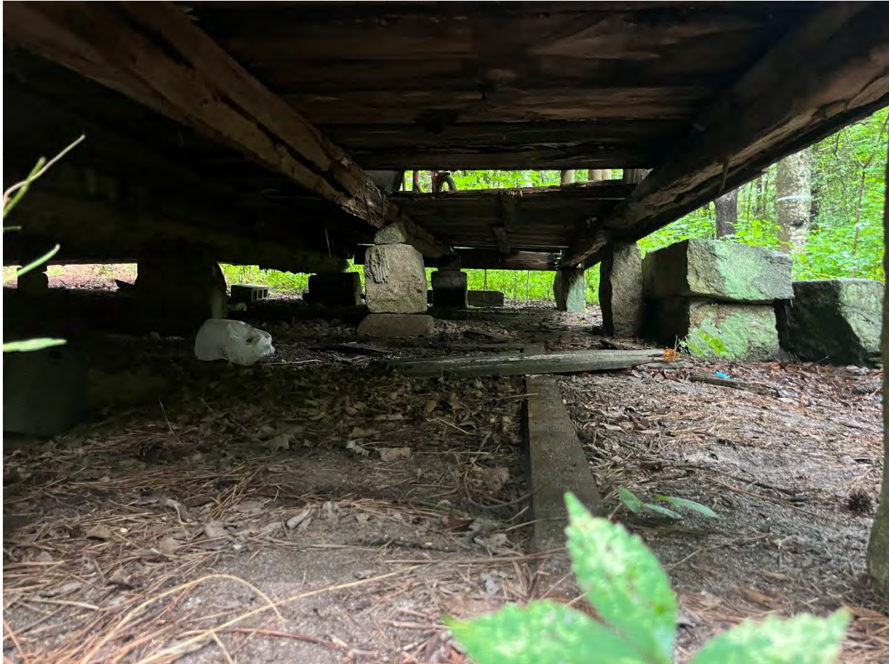
Photo 10 – Floor Framing and Rock Supports
