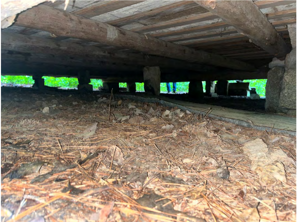
Photo 9 – Floor Framing and Rock Supports
