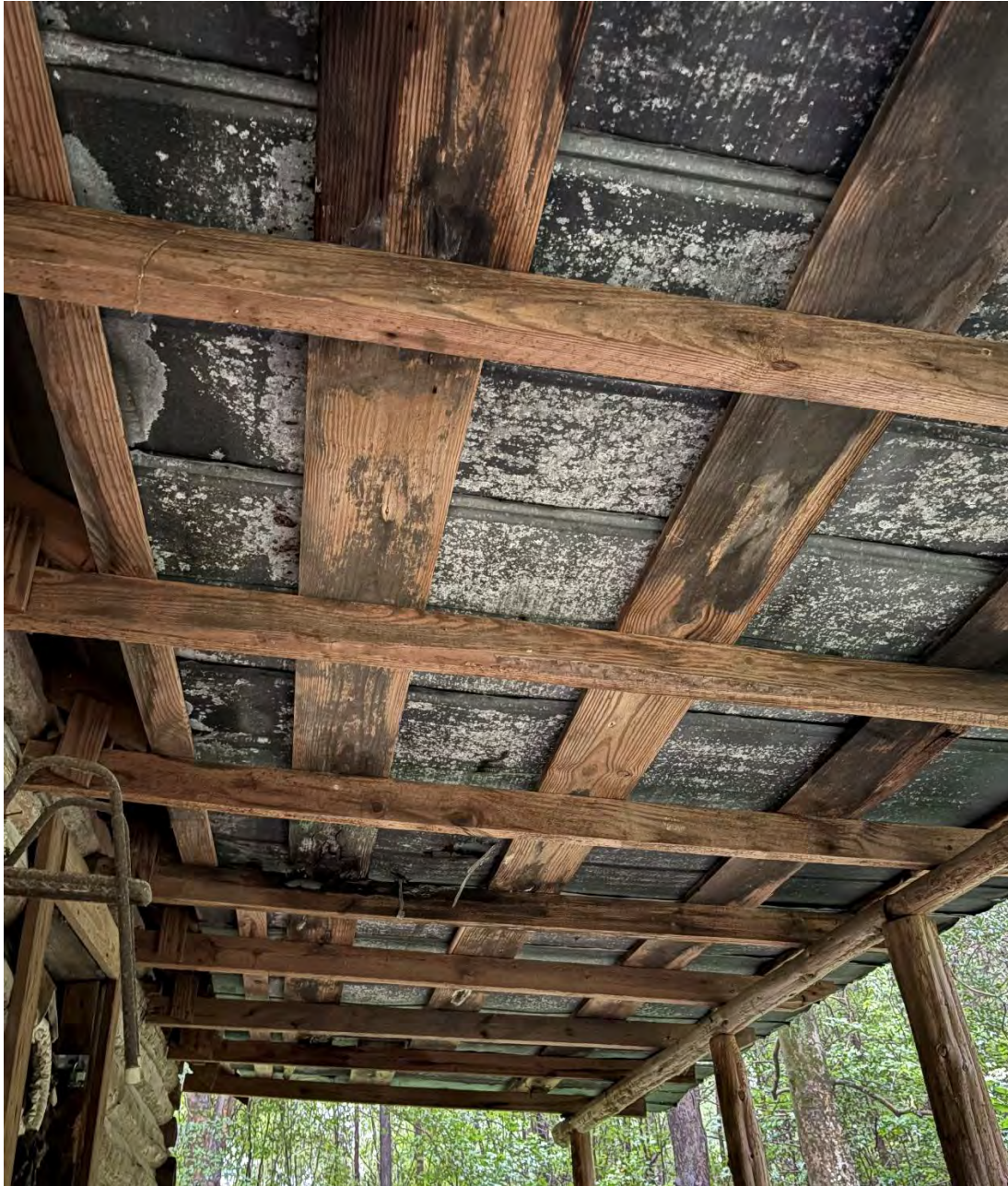
Photo 7 – Porch Roof Framing
