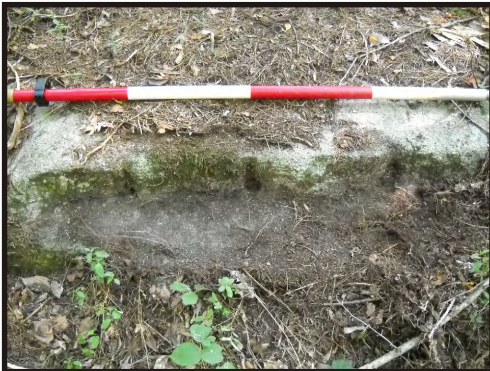
View of quarrying activity to west of 31WA1772/1772**. Note three drill holes.
