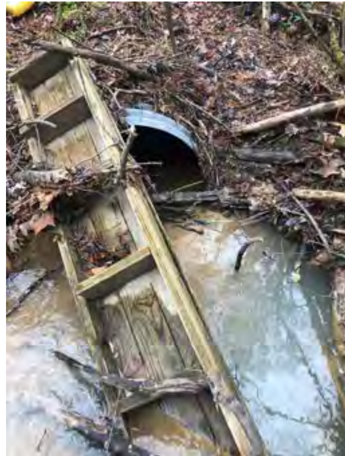
Culvert under Oak Hill Drive roadbed
