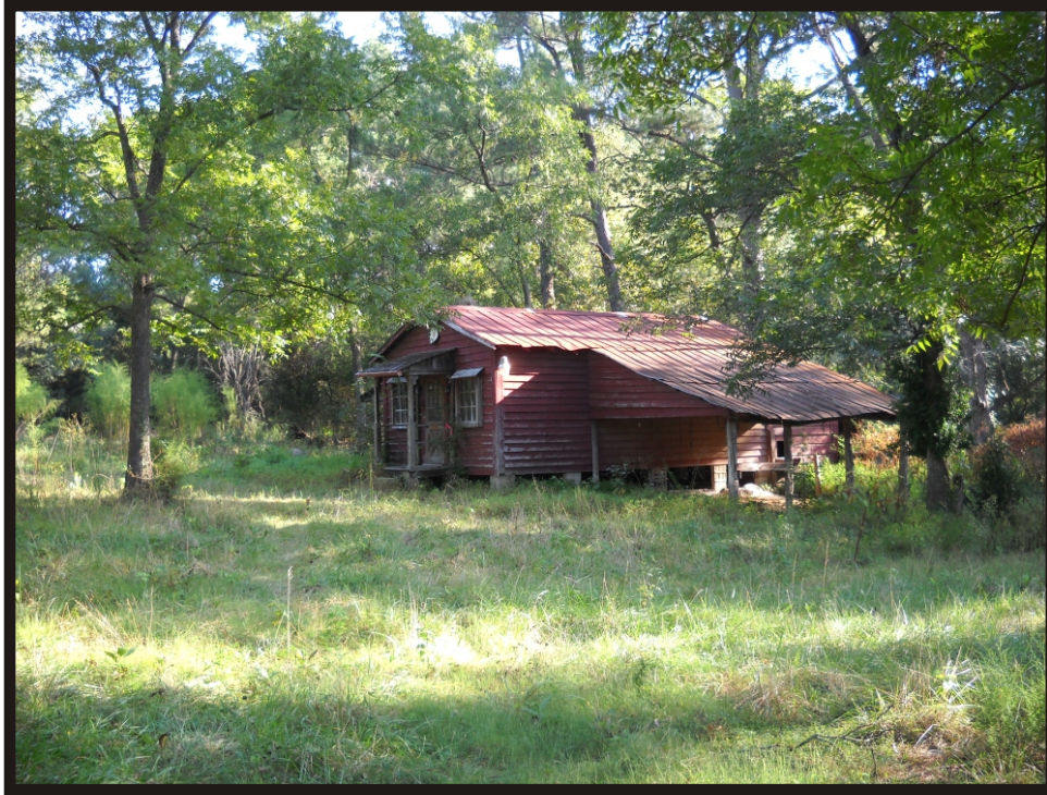
View of red barn in northeast portion of 31WA1773/1773**, facing northeast.
