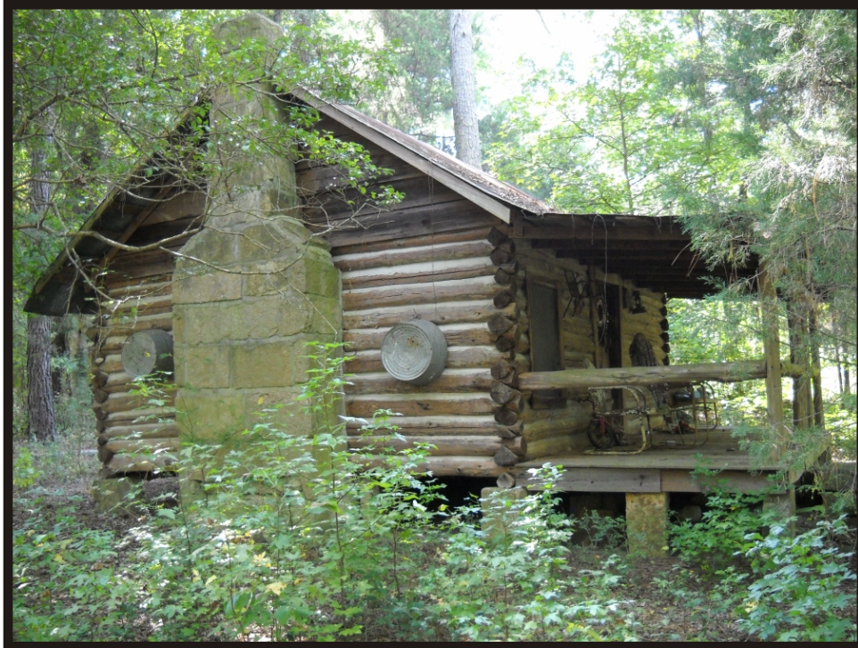
View of north and west elevations of cabin, facing southeast.
