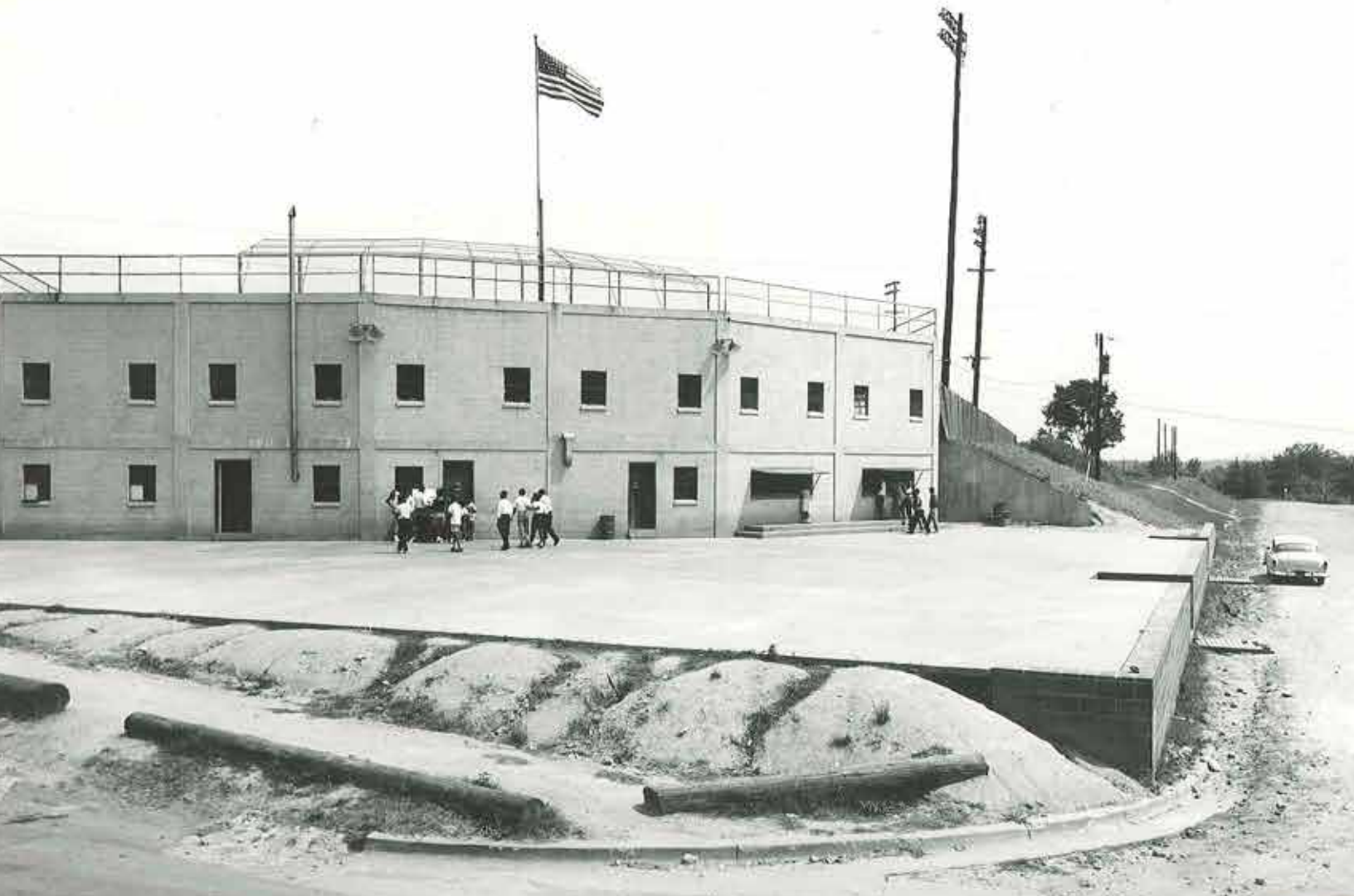
Grandstand and Stadium Entrance | Source City of Raleigh Parks, Recreation and Cultural Resources, Digital Files
