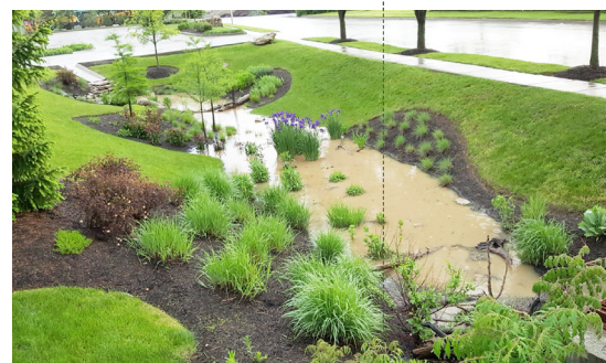
07 GREEN STORMWATER INFRASTRUCTURE
