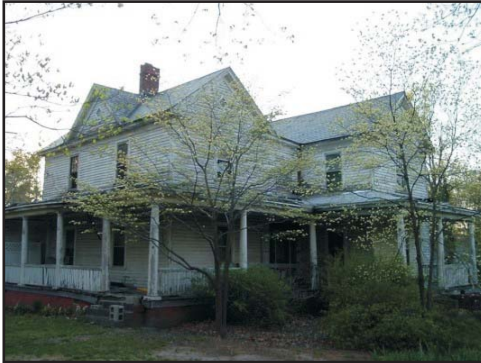
South and east elevations.
