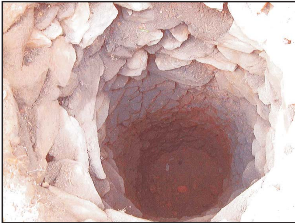
View down well prior to being capped with concrete slab.
