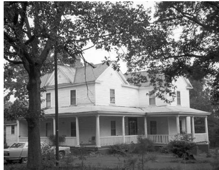
Latta House ca. 2006 Photo Credit: NC State Archives
