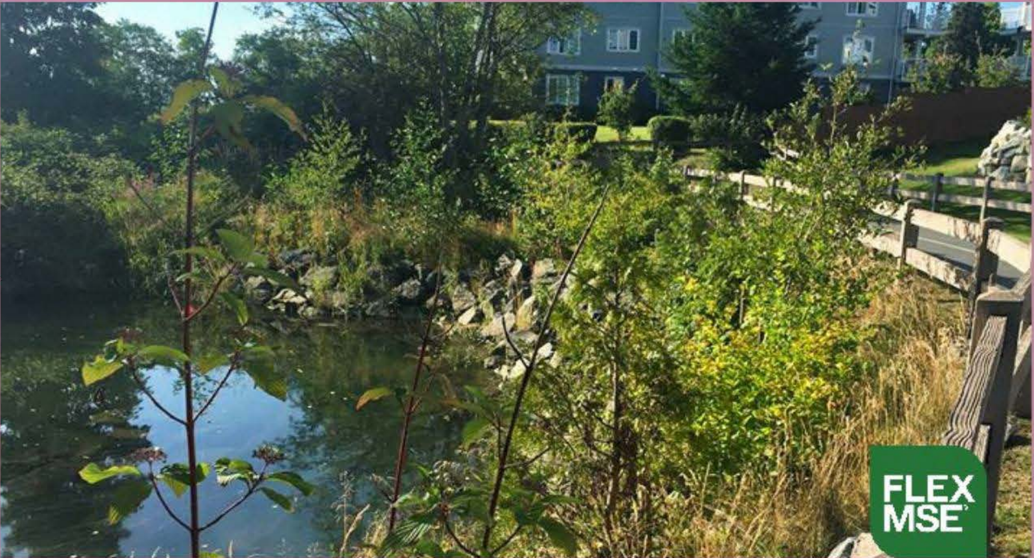
Reinforcing the stream bank with materials and native plants to prevent erosion
