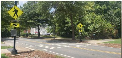
RRFB - Rectangular Rapid Flashing Beacon
