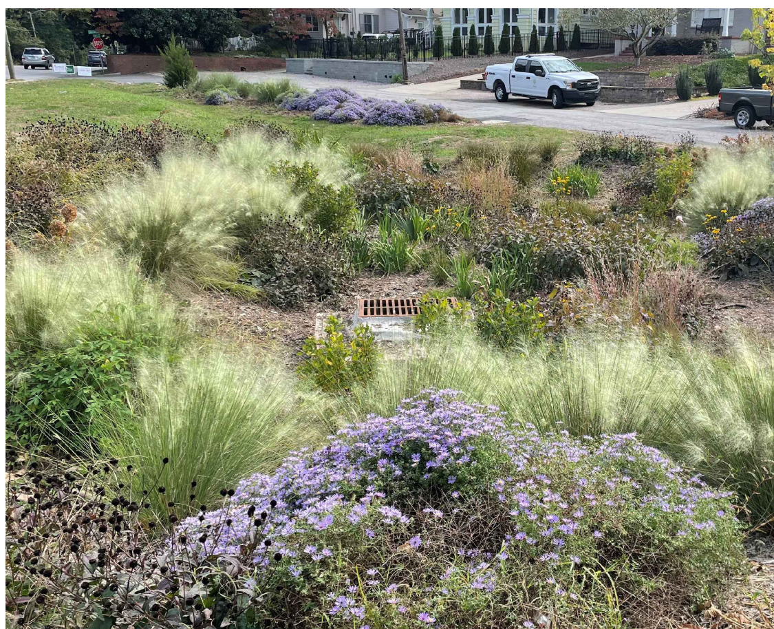
RAIN GARDEN (GREEN STORMWATER INFRASTRUCTURE)
